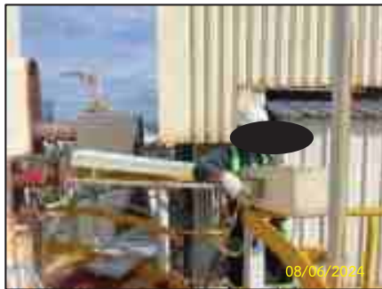
(ก) Recovery Boiler Stack
